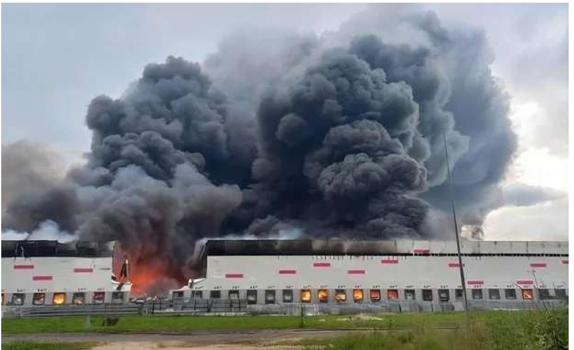
Smoke rises as firefighters work to extinguish a fire at a Wildberries logistics hub following a Ukrainian drone attack in Russia's Ryazan region.
